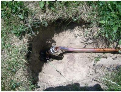
I drilled the pipe into the ground until the pipe top was ~6" below the surface of the ground. I used two Vice-Grip's<sup>TM</sup> pliers as handles onto the copper pipe. I work the pipe up and down allowing the water to flush the soil and small gravel from the pipe tip. If you hit a rock – pull it out and change the attack angle slightly and re-drill. The feature of hydra-drilling is if you need to pull out the pipe the water pressure will help you and keep the hole lubricated – easy work.
