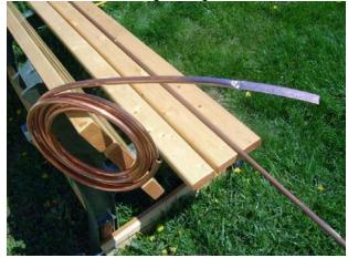
The soft copper tubing is buried at least 6" deep. This will keep you from hitting the ground system with the lawn mower or becoming a trip hazard. The buried copper tubing will also add to your energy dissipating ground system. Burying the bare copper tubing insures maximum "ground system" conductivity is obtained with an additional benefit by watering your lawn you will increase near surface soil conductivity - a HINT during contesting.
